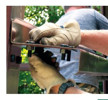
Engineered cees and zees **bolt together** with solid steel plates to give its strength.
