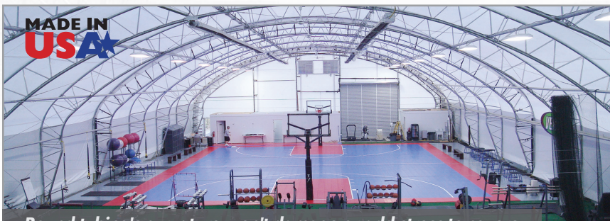
Round tubing's curvature won't damage or add stress to covers.
